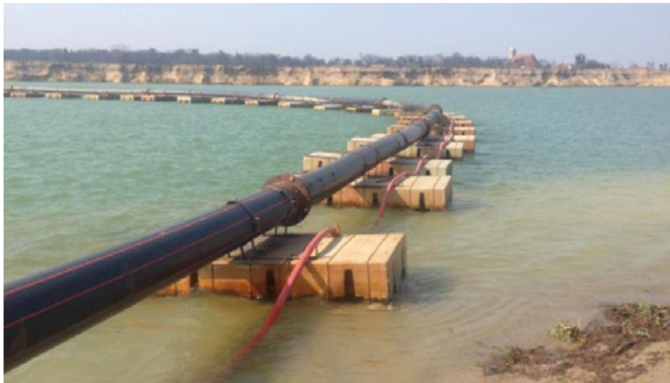
An exemplary application of W-series single floats for hydrotransport pipe.
